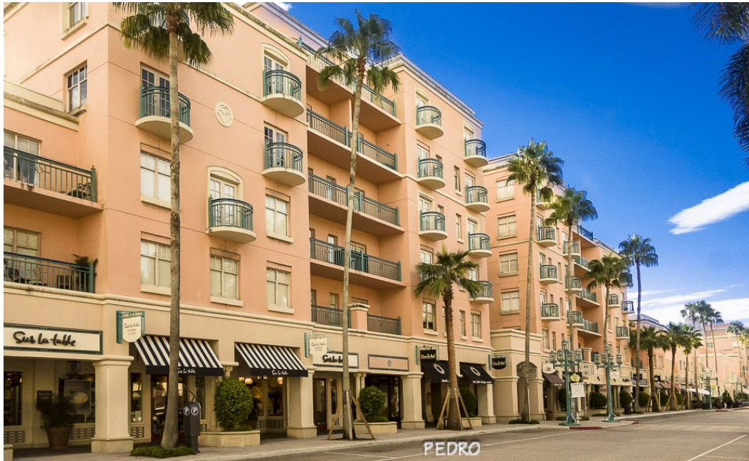
Mizner Park, Boca Raton, FL - 29 Acres – 3 to 6 Stories - Commercial/Office/Amphitheater; 272 Residential Dwelling Units
