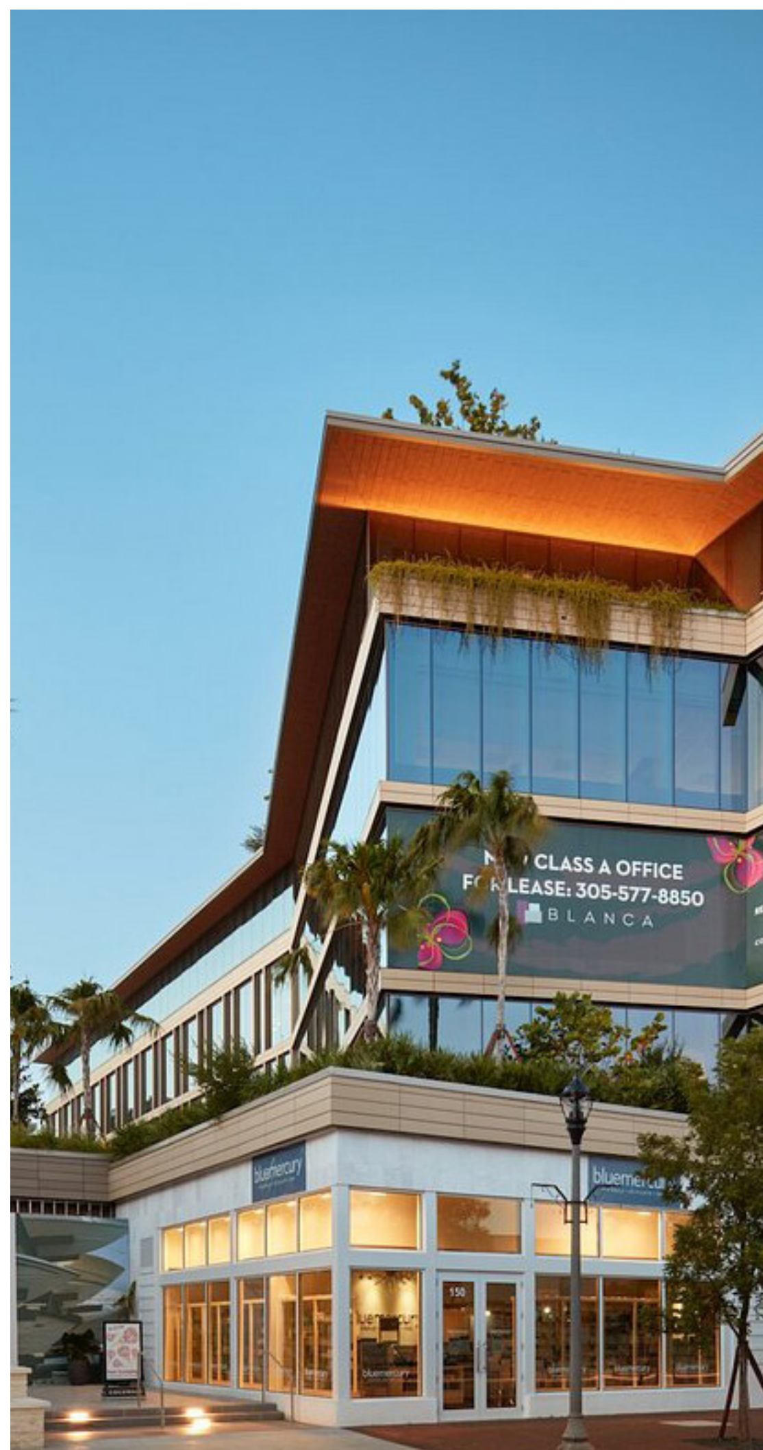
Mixed-use buildings maintain a higher percentage of glazing (US1 and Sunset Place).
