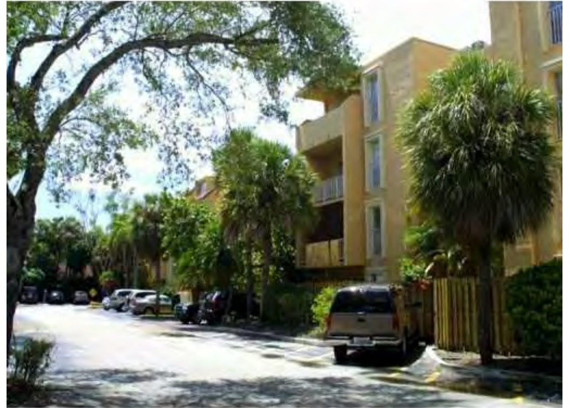
Dadeland Grove Apartments: 34 du/acre
